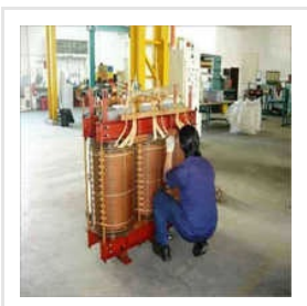
Power Transformer Repairing Services
