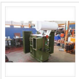
Distribution Transformer Repairing
