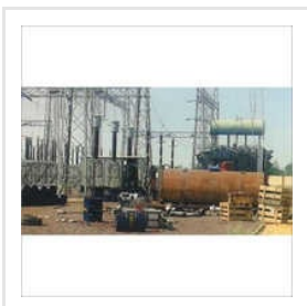
Sub Station Transformer Repairing
