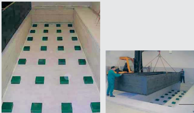
Application example in the plant of a major automobile manufacturer. Passive insulation protection of a Waldrich-Coburg portal milling machine from the pressing mechanism sector. Total mass: approx. 1200 to.
