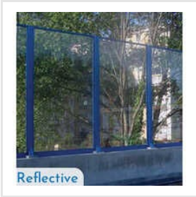
Reflective Noise Barrier
