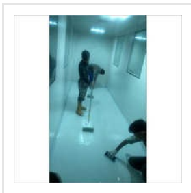
Epoxy Screeding Service
