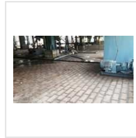
Acid Proof Tiles Silicate Installation Service
