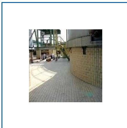
ACID PROOF BRICK LINING SERVICES
