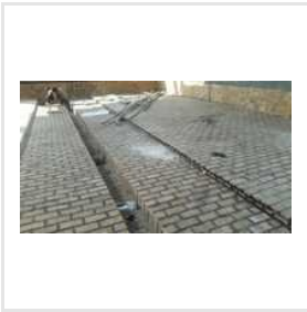
Acid Proof Tiles Lining Work
