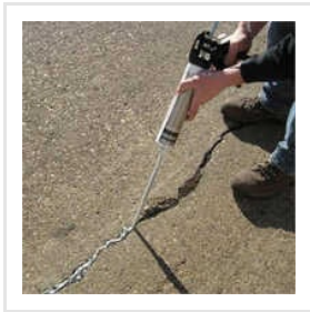
Epoxy Crack Filling Service
