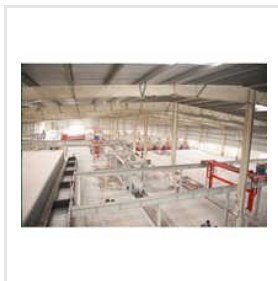
Autoclaved Aerated Concrete Plant
