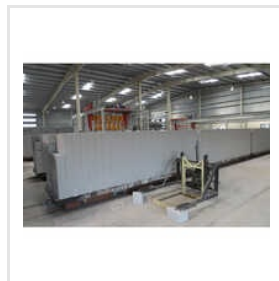
Big AAC Block Plant
