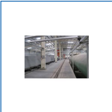
SMALL AAC PLANT
