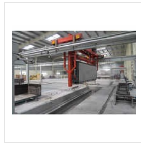
AAC Panel Plant
