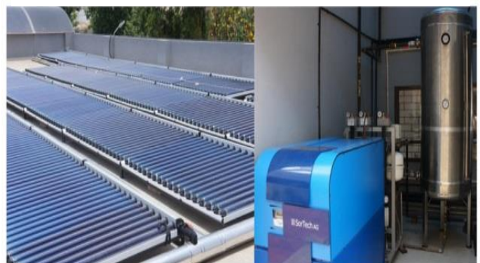
Central Solar Air Conditioning System
