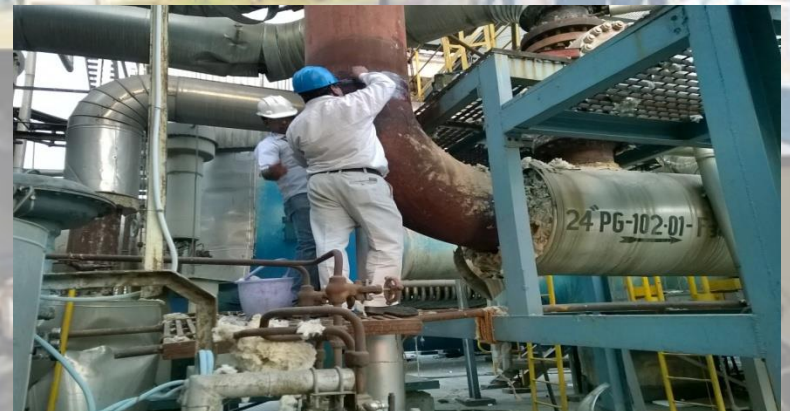
Ultrasonic Testing of critical pipeline being carried out
