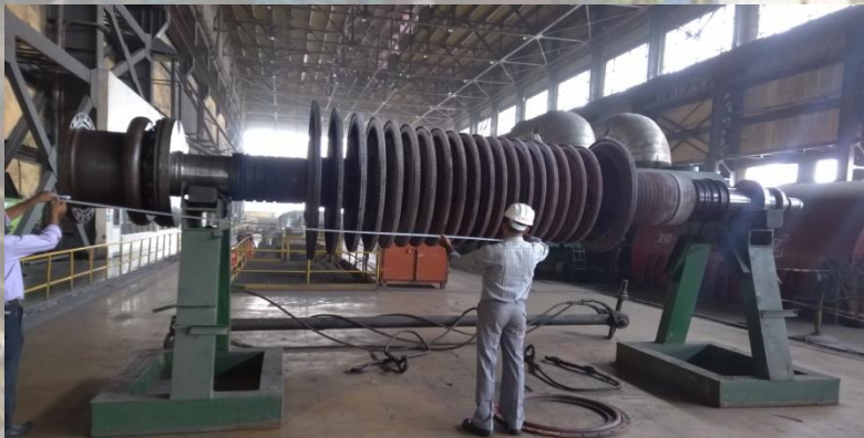
LP Stage of 95 MW unit being inspected for flaws
