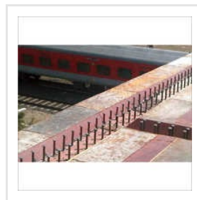
Rail Over Bridges And Girders Welding Stud
