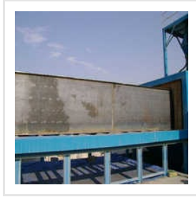
Structure Shot Blasting
