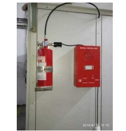
Direct Fire Suppression System
