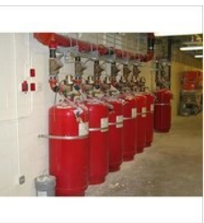
Fire Suppression System For Server
