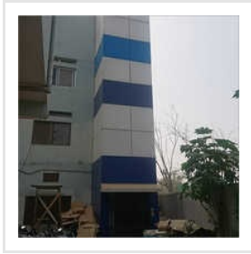
Industrial Goods Elevator
