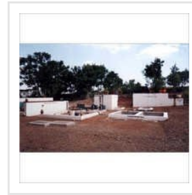
Industrial Sewage Treatment Plants
