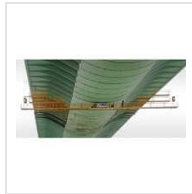
Hoisting Hanging Rope Platform
