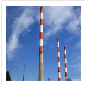
Fabricated Industrial Chimney
