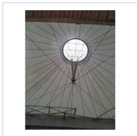
Industrial Tensile Canopy Structure
