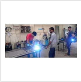
Welding And Fabrication Service
