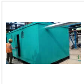
Engine Acoustic Enclosure
