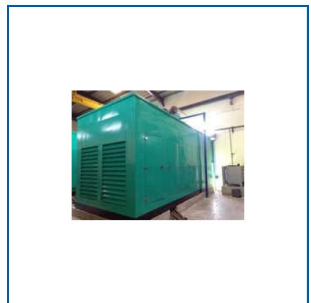
DG SET ACOUSTIC ENCLOSURE
