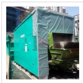
Concrete Pump Acoustic Enclosure
