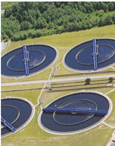
Waster Water Treatment
