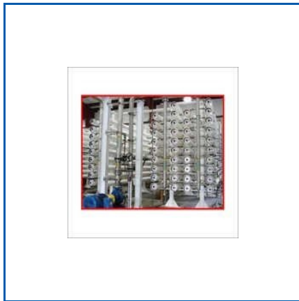
RO MEMBRANE PLANT SERVICES
