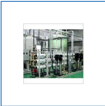
RO PLANT REPAIRING SERVICES
