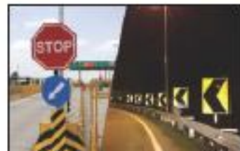
Hazard Marker & Chevron Sign Boards
