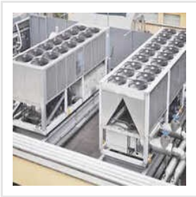
HVAC System Service
