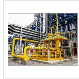
Nitrogen Piping And Plant Relocation
