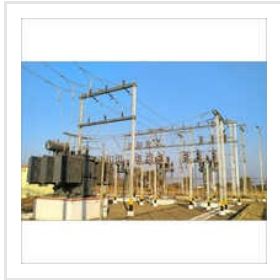
HT Substation Work Service
