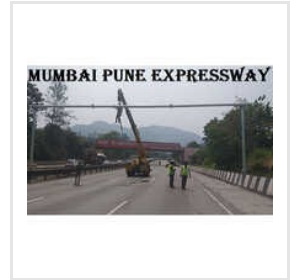
16 Mtr NS Gantry Installation Services
