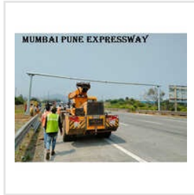
Gantry Poles Installation Services
