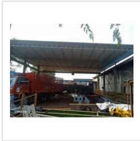
Industrial PEB Structure Shed
