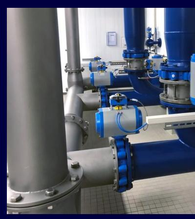
VB Series rack and pinion actuators are designed to automate the most popular quarter turn valves like ball, butterfly and plug valves and are easily adaptable for almost any other quarter turn (90° rotation) application.
