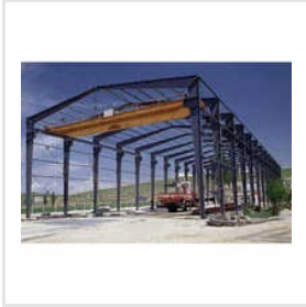
Pre Engineered Steel Building Structure
