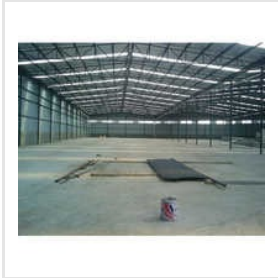
Pre Engineered Building
