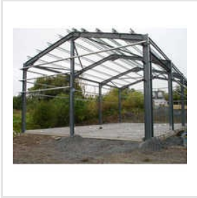
Prefabricated Metal Structure
