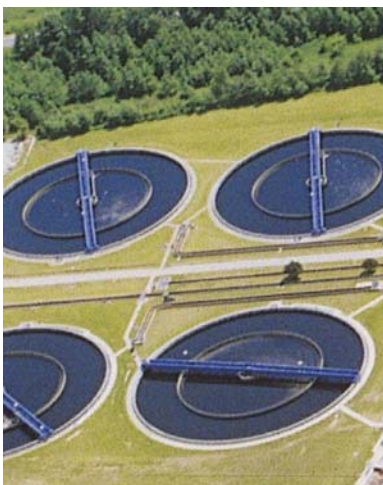
Waster Water Treatment
