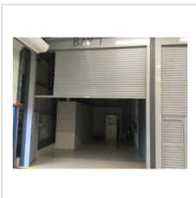
Motorized Rolling Shutter Fabrication
