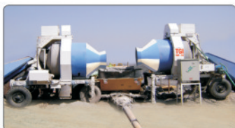
FEEDING TO CONCRE PUMP
