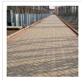
Anchor Boulevard Paver Block
