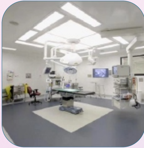
Hospital Operation Theatre
