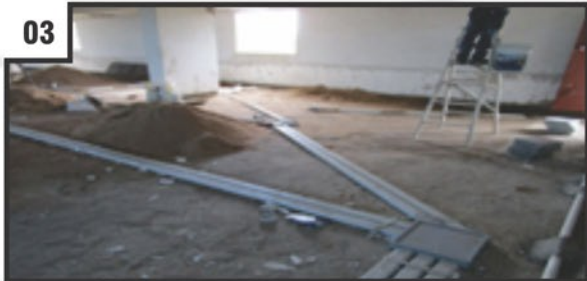
Trunking, electric and networking and other wall furnishing work.
