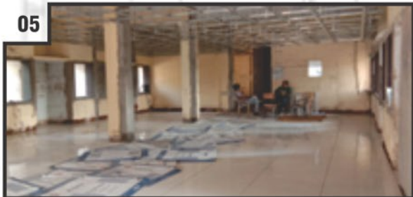
Finished flooring and false ceiling structure.
