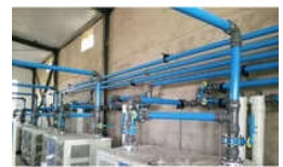
Industrial Compressed Air Pipeline
