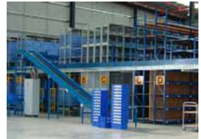
GB - 197 Mezzanine Floor racking system
