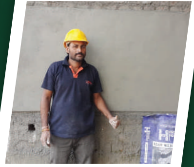
Govt Project (Jhs)
