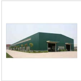
PEB Industrial Shed
