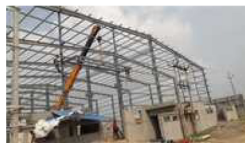
PEB Structure Industrial Shed
