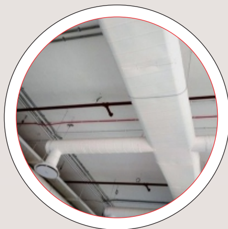
Double Wall Spiral Flat Oval Duct
