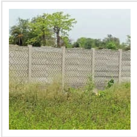
Precast Compound Wall
