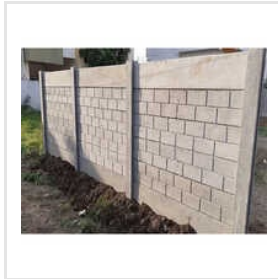
Concrete Boundary Wall
