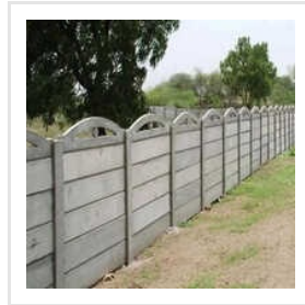
Concrete Compound Wall
