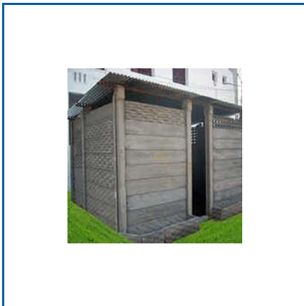
SECURITY ROOM WITH WALL
