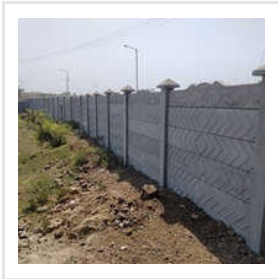
RCC Boundary Wall
