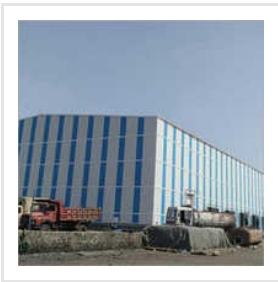
PUF Cold Storage
