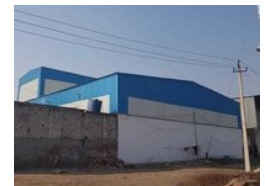
Rafter System Building
