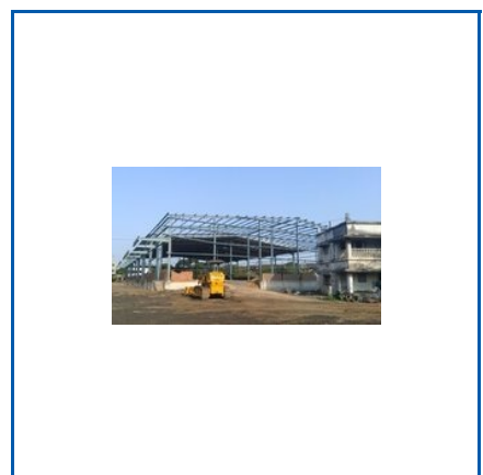
METAL BUILDING CONSTRUCTION FOR INDUSTRIAL
