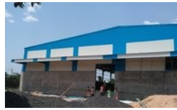
Workshops Building Structure
