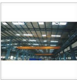
Pre Engineering Building With Cranes
