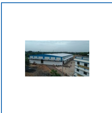
PRE ENGINEERED BUILDING
