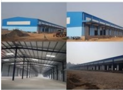
Prefabricated Steel Shed
