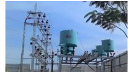
Harmonic Filter Reactor
