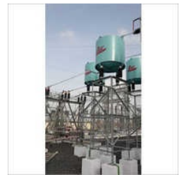
Current Limiting Reactor
