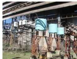
Harmonic Filter Reactors
