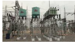
Air Core Reactor
