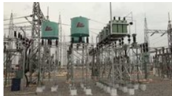
33 KV Capacitor Bank
