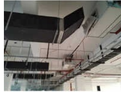
Air Ducting Execution Project
