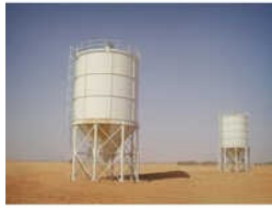
Bolted Cement Silo
