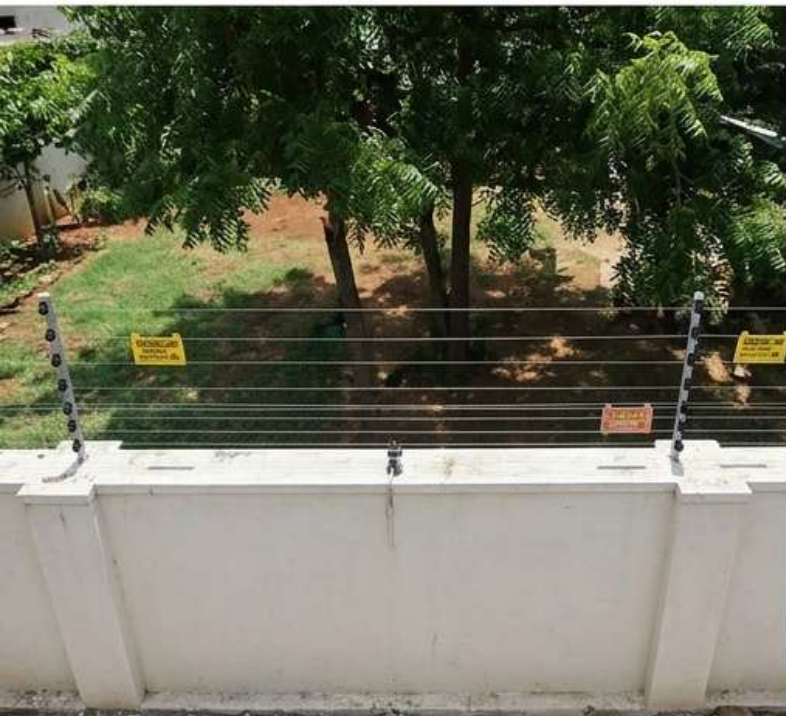
View 3: Wire & Insulator Detail
