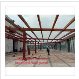
Structure For Puf Insulated Roof Panel
