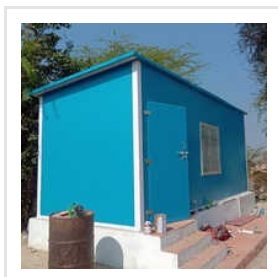
RO Plant Shelter
