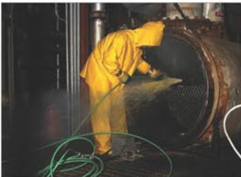
Tube Cleaning - Internal
