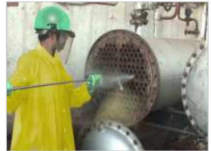
Power Plant Condenser Tube cleaning
