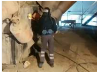
Pre Heaters Cleaning
