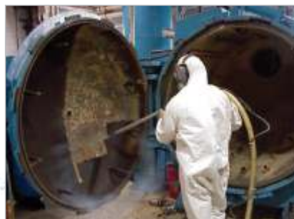
Cement Silo Cleaning
