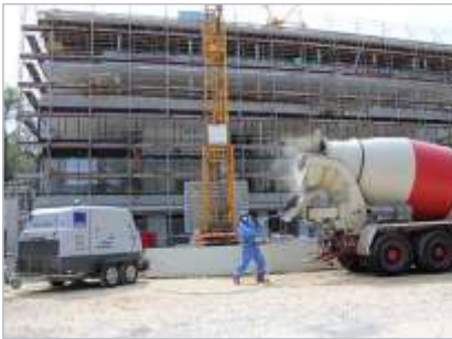
Ready Mix Concrete Truck Cleaning
