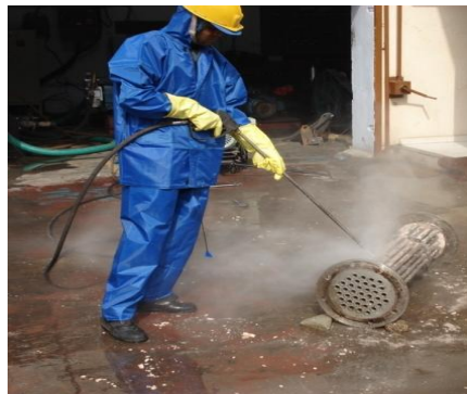
Tube Bundle Cleaning – External
