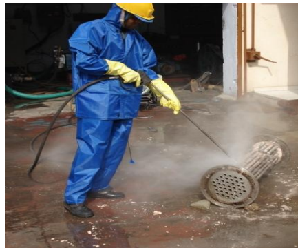
Tube Bundle Cleaning – External
