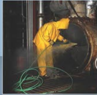
Tube Cleaning - Internal
