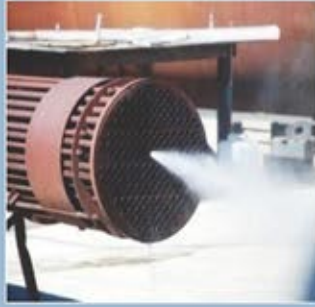
Internal Tube Cleaning
