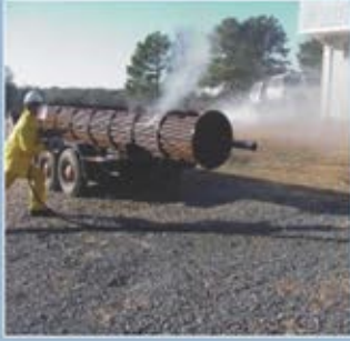
External Tube Bundle Cleaning
