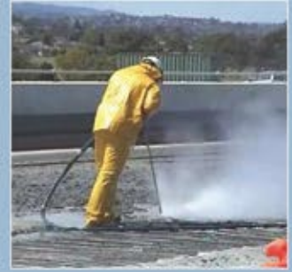
Concrete Removal
