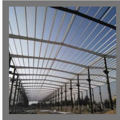
Steel Shed Shelter
