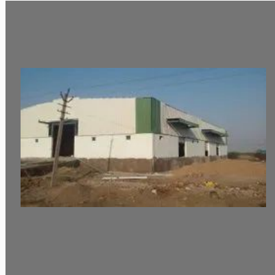
Peb Warehouse Shed
