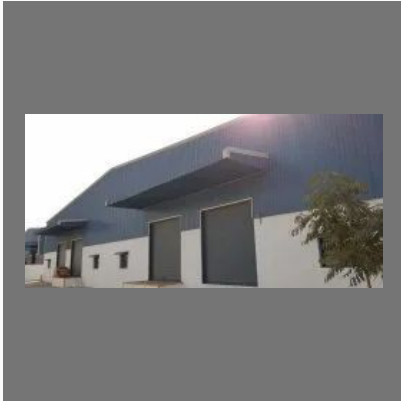
Warehouse Construction Services
