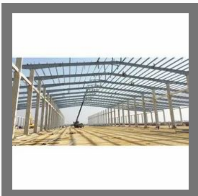
Prefabricated structure in mumbai
