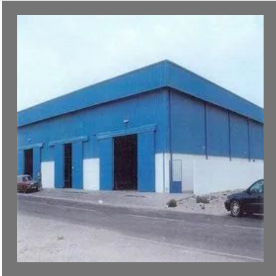
Industrial Shed Fabrication
