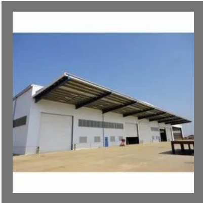
Mild Steel Industrial Warehouse Shed
