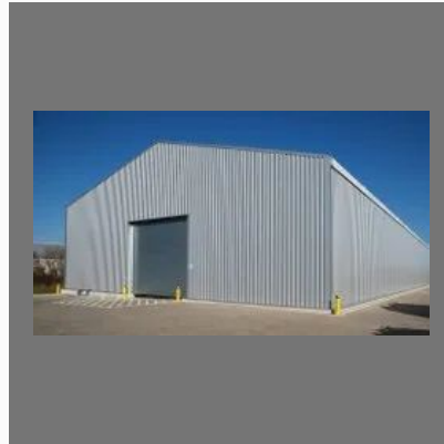
Mild Steel Industrial Warehouse Shed
