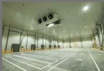
Cold Storage Structure
