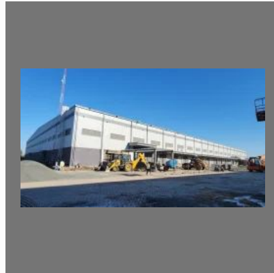
Industrial shed construction
