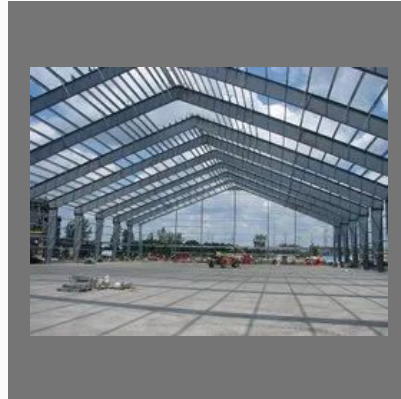
Pre Engineered Building Structure
